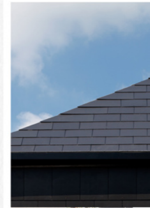
③ natural slate tiles
